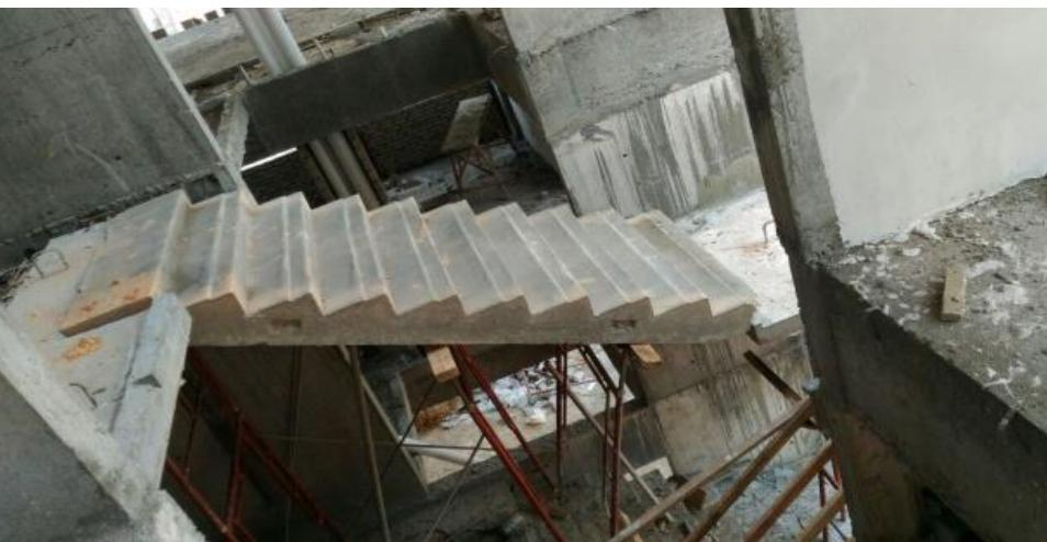
IBS Staircases and Landing Slab Installation
