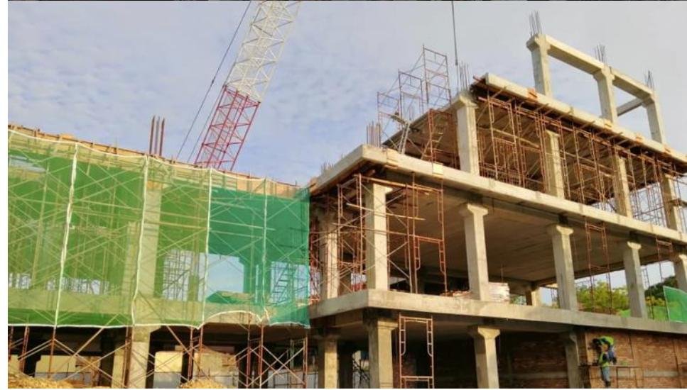
IBS Precast Installation (Column, Beam and Half Slab)
