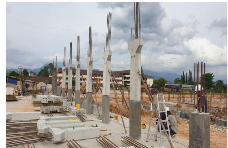
IBS Precast Installation (Column, Beam & Hollow Core Slab)
